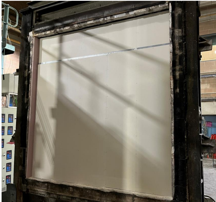
Photo 5 -Third layer of boarding on the exposed side
