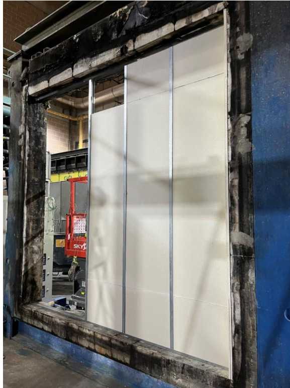
Photo 1 - Specimen During construction – Exposed side
