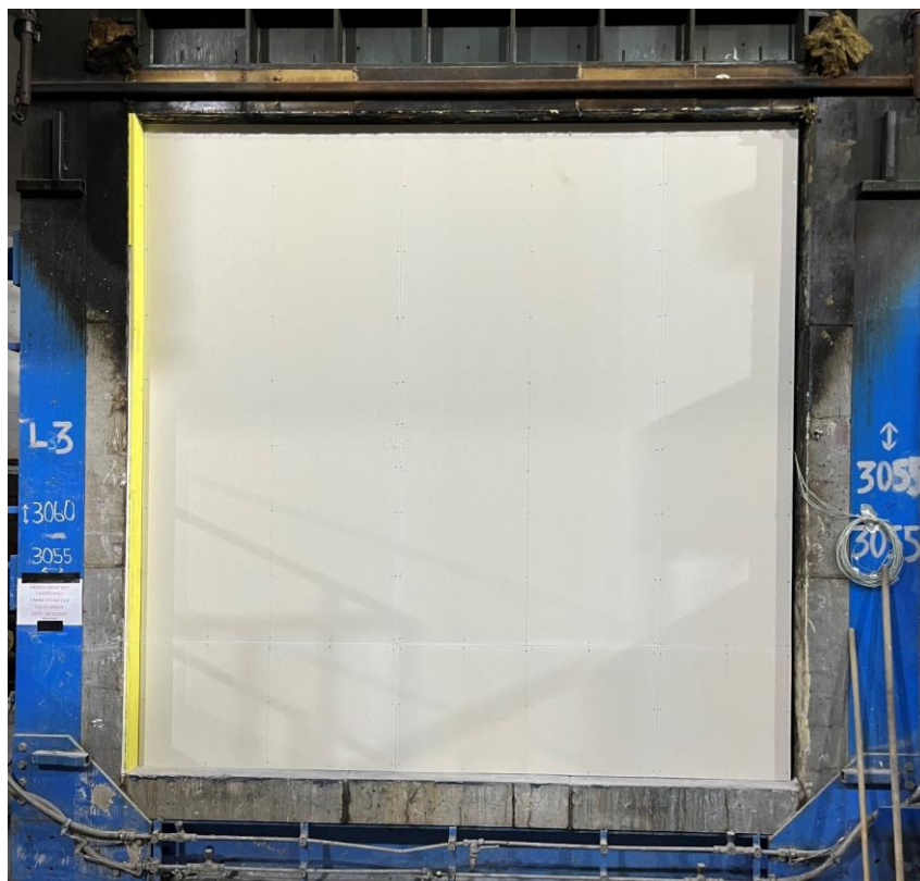
Photo 4 – Second layer of boarding on the unexposed side
